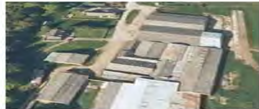
photo below: redundant and dilapidated sheds set against Culloden Wood and "Viewhill" (source: Google)
