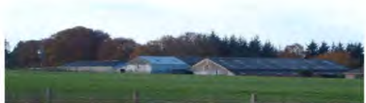
photo above: looking north-west: the existing bulk agricultural buildings 6.5m - 9.0 m high, open foreground and backdrop of tall trees
